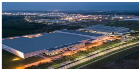
Premium Electrical SubStation
